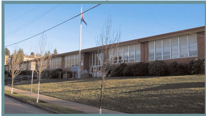
Mt. Tabor Middle School 5800 SE Ash Street Portland, OR 97215
